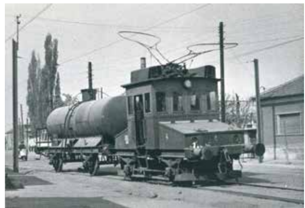
Fig. 13. Electrical locomotive built in Oradea, on service on Calea Clujului (around 1974)
